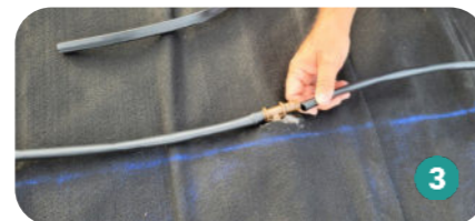
Before cutting, make sure the pipes for the drip irrigation have been drawn from the roof ridge.
