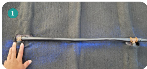
Before cutting, make sure the pipes for the drip irrigation have been drawn from the roof ridge.
